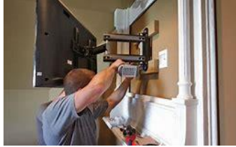
Installation of TV, mounting kit
